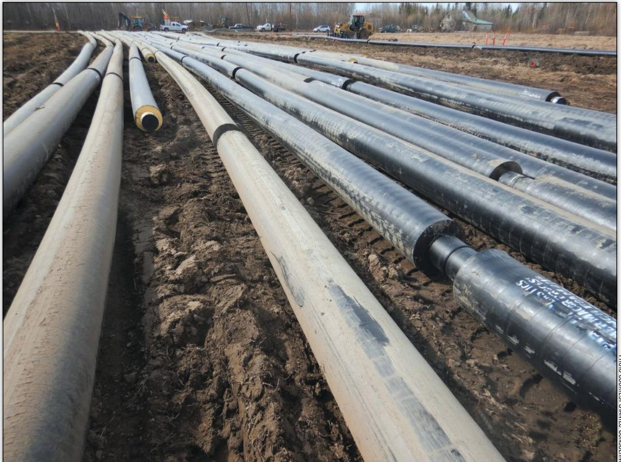
Stantec Consulting played a key role in installing the North Pole Water Expansion project, which includes more than 34 miles of high-density polyethylene pipe. The project was completed in September 2019, three months ahead of schedule.
