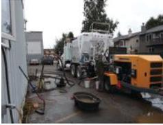
Compaction grouting equipment injecting low-mobility grout to stabilize poor soils and raise the foundation.
