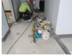
Slabjacking interior floor with cellular concrete after earthquake.
